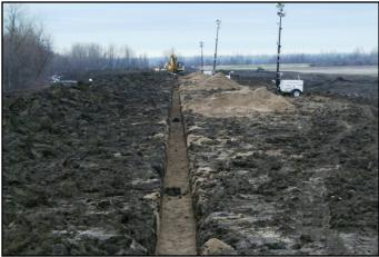
Contractors install pipes as part of the operating system for the Floodway levee. This is one of the final steps leading to the full restoration of the frontline levee.
